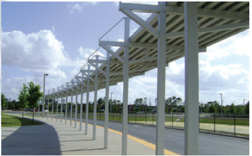
RIGHT: LAWTON CHILES MIDDLE SCHOOL OVIEDO, FL ARCHITECT: SCHENKEL SHULTZ ELKINS CONSTRUCTORS
