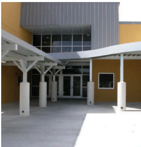
LEFT AND BELOW LEFT: CYPRESS PALM MIDDLE SCHOOL NAPLES, FL ARCHITECT: FAWLEY BRYANT OWEN AMES KIMBALL
